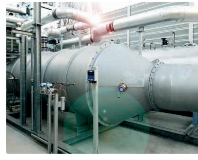
Incineration provides a safe option for the destruction of liquid and gaseous waste as well as the recovery of process heat generated to produce hot water, thermal oil, hot air or steam. Each incinerator plant is customized to our client's needs. Especially with respect to our customer's waste management, ensuring savings on transportation, simplifying the handling of waste and increasing the waste reduction efficiency.
