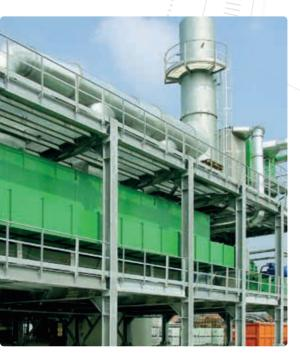
Under specific conditions of high mono- or bi-solvent concentration, the use of activated carbon is suitable for the internal regeneration process after being saturated with organic substances.
