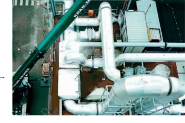
Nitrogen oxides  $NO_X$  are removed by a Selective Catalytic Reduction composed of an active catalyst operating in combination with injected ammonia or urea into the process gas. This converts the nitrogen oxides (NO and NO<sub>2</sub>) to nitrogen (N<sub>2</sub>) and water (H<sub>2</sub>O). The required performance can be achieved at low temperatures, supporting the overall energy reduction program of the facility.
