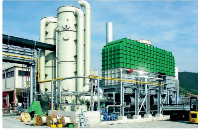
**Airprotech** assures the high destruction efficiency of pollutants in a safe and controlled environment, ensuring an effective combustion chamber temperature and residence time suitable for the complete oxidation of halogenated compounds. In addition, specialized engineering of **Airprotech** plants ensures high reliability and resistance to aggressive substances over time.
