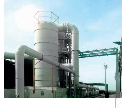
Scrubber Solutions may only be with water for water-soluble substances or solutions with reagents that specifically target certain inorganic compounds to be neutralized. The design of the plant and the choice of the chemical reagent depends on the substances contained in the gas to be purified.
